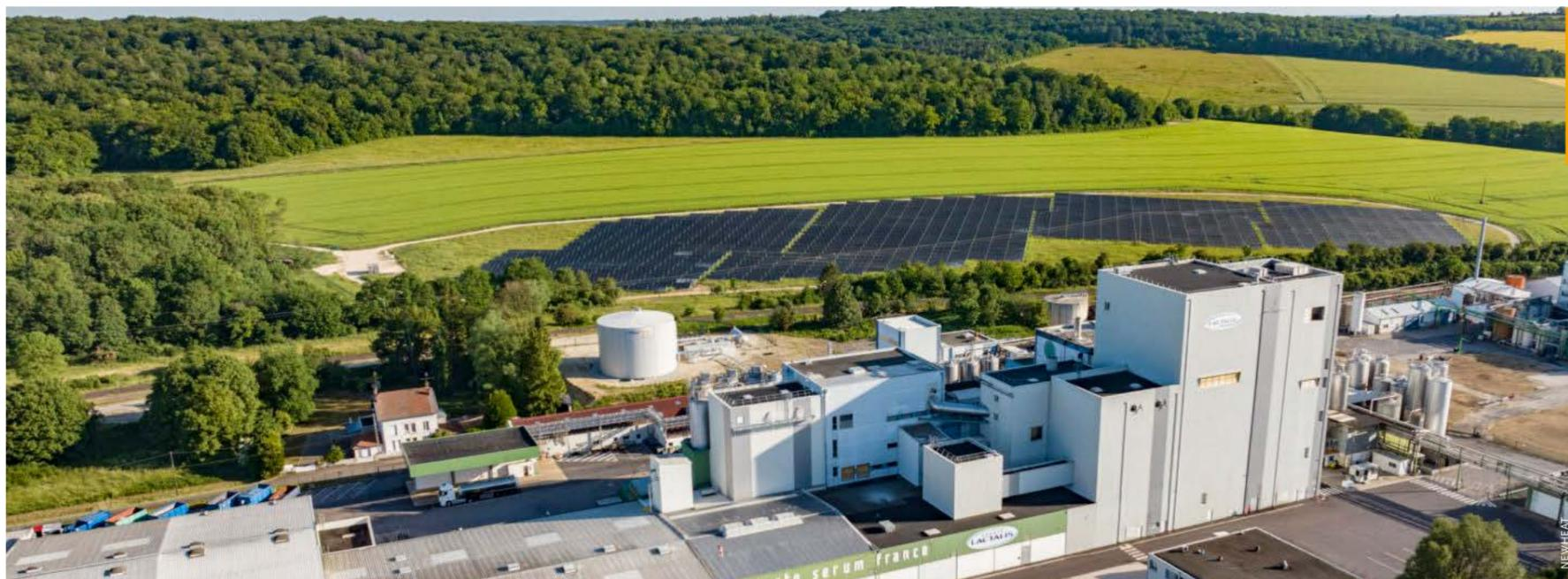
*The power plant of the French Lactalis group's whey powder plant at Fromeréville-les-Vallons near Verdun. The plant has a 15 300-m<sup>2</sup> field of solar thermal collectors which provide 14 MWth of solar capacity and is equipped with a 3 000-m<sup>3</sup> hot water storage system.*
