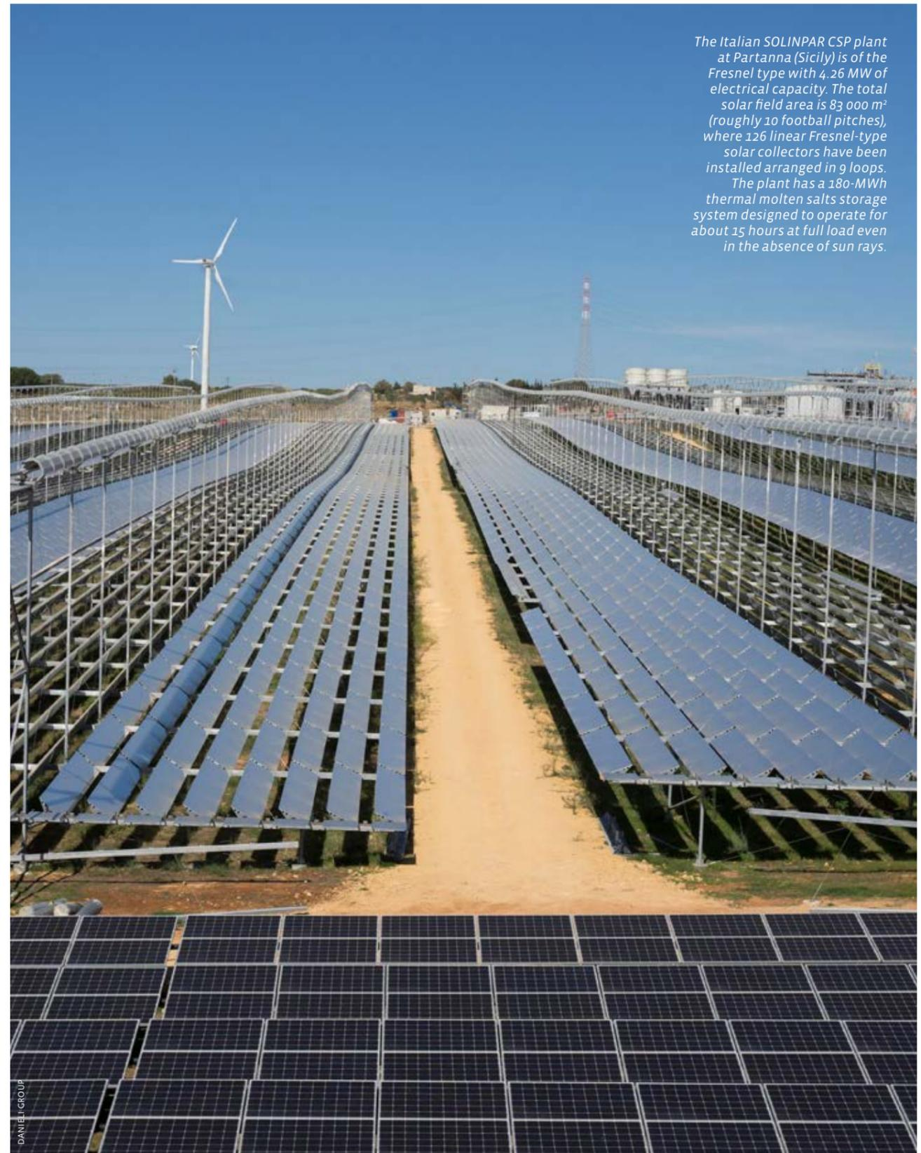
The Italian SOLINPAR CSP plant at Partanna (Sicily) is of the Fresnel type with 4.26 MW of electrical capacity. The total solar field area is 83 000 m<sup>2</sup> (roughly 10 football pitches), where 126 linear Fresnel-type solar collectors have been installed arranged in 9 loops. The plant has a 180-MWh thermal molten salts storage system designed to operate for about 15 hours at full load even in the absence of sun rays.
