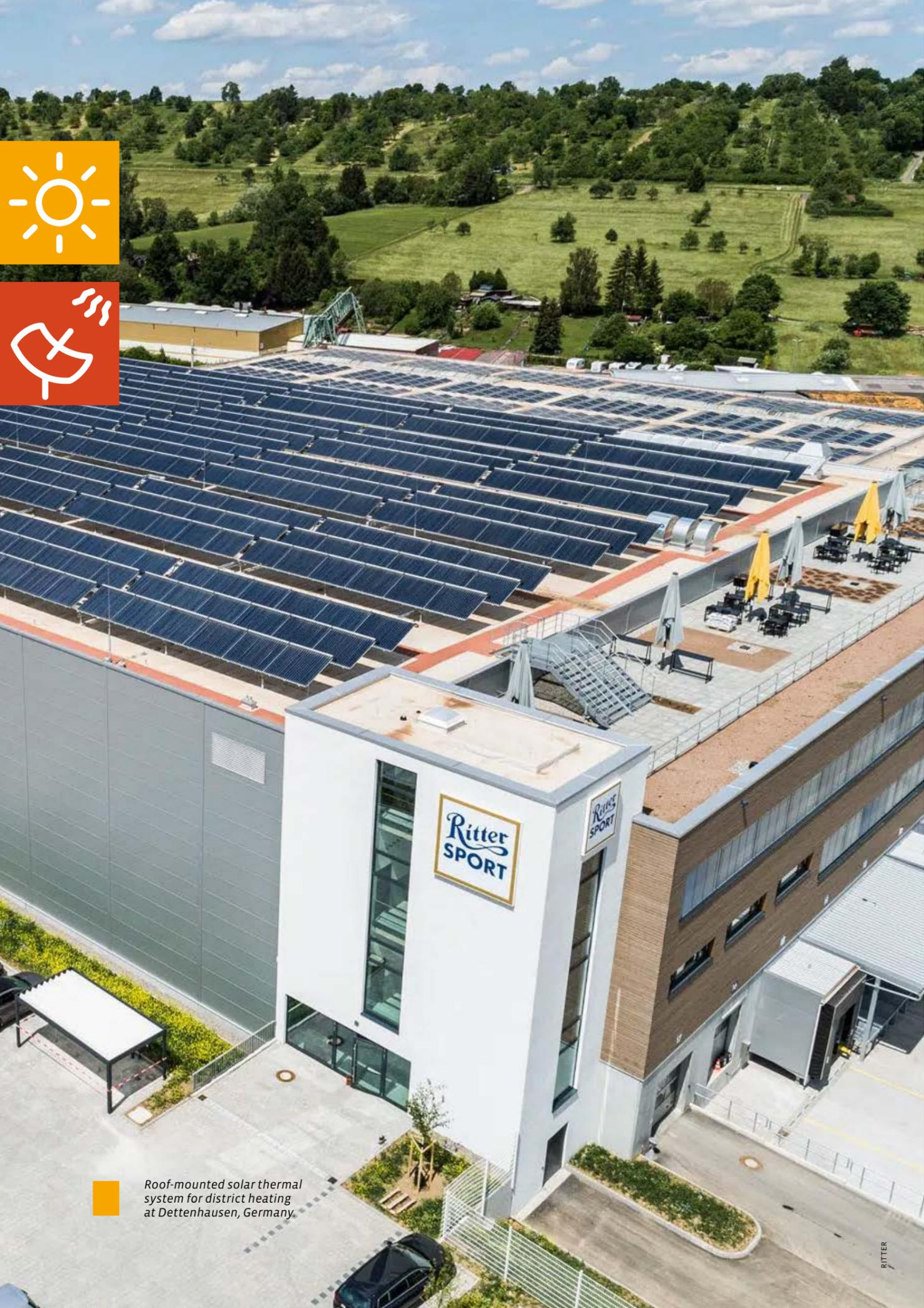
Roof-mounted solar thermal system for district heating at Dettenhausen, Germany.
