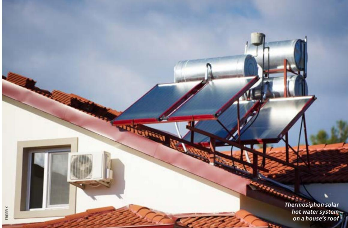
Thermosiphon solar hot water system on a house's roof
