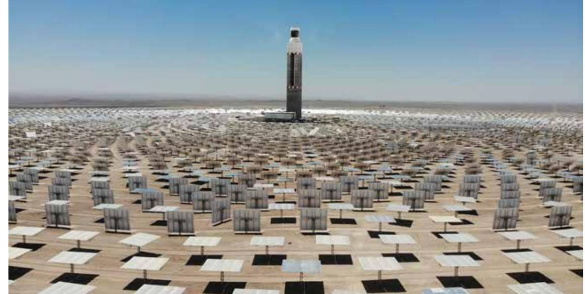
latter, with its 600 MW of capacity and 11-hour storage system, will take CSP technology into a new era.
