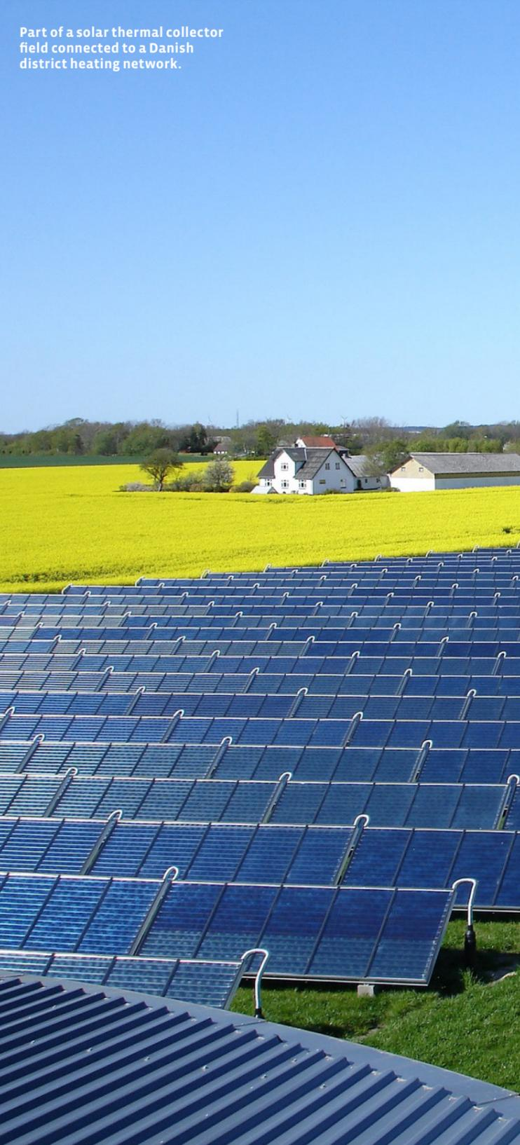
Part of a solar thermal collector field connected to a Danish district heating network.
