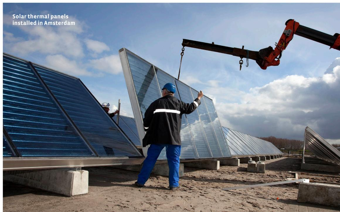
Solar thermal panels installed in Amsterdam
