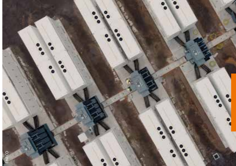
In February 2025, Eneco, Belgium's green electricity supplier, started up the country's biggest battery storage park at Ville-sur-Haine. The site can now store up to 50 MW/200 MWh of energy, which equates to 4 hours of energy on the high voltage grid.
