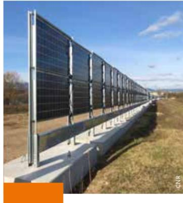
The Compagnie nationale du Rhône (CNR) has commissioned a demonstrator with vertical bifacial modules on the Sablons dyke (Isère). It is deployed over 350 metres with 104 kW of installed capacity. These 3-metre high panels are more resilient and watertight than classic ground-based PV panels.
