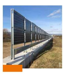
The Compagnie nationale du Rhône (CNR) has commissioned a demonstrator with vertical bifacial modules on the Sablons dyke (Isère). It is deployed over 350 metres with 104 kW of installed capacity. These 3-metre high panels are more resilient and watertight than classic ground-based PV panels.
