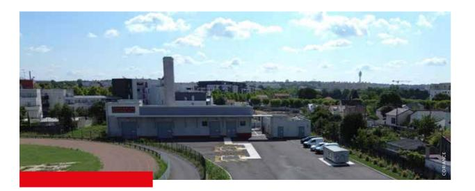
In September 2024, a second geothermal district heating network was inaugurated in Champigny-sur-Marne, (Île-de-France). According to its operator, Coriance, Champigny 2 has a geothermal capacity of 16 MWth—the same as Champigny 1—supplemented by a 2.2 MW heat pump. Construction. which began in 2022, included 9.2 kilometers of piping and two wells drilled to a depth of 1800 meters into the Dogger formation (69.4 °C; 350 m³/h).
