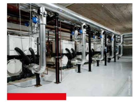
The geothermal project in the Pleyel district of Saint-Denis, in the Paris region, involves drilling 11 shallow geothermal wells equipped with reversible heat pumps and extending the existing heating network by 10 kilometres. The system will provide an annual heat supply of up to 30 MWh and a cooling supply of up to 10 MWh to the new urban district created from the conversion of the Olympic and Paralympic Village, the future Pleyel ZAC, as well as the Pleyel Tower, now converted into a hotel.
