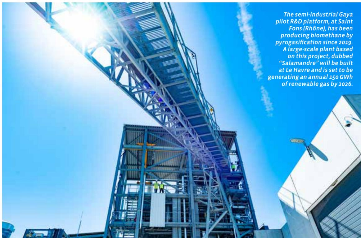
The semi-industrial Gaya pilot R&D platform, at Saint Fons (Rhône), has been producing biomethane by pyrogasification since 2019. A large-scale plant based on this project, dubbed "Salamandre" will be built at Le Havre and is set to be generating an annual 150 GWh of renewable gas by 2026.
