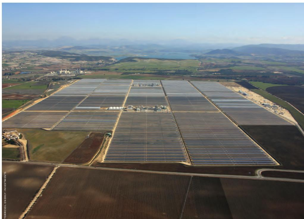
**C**oncentrated solar power covers all the technologies harnessed to transform the energy radiated by the sun into very high temperature heat. This thermal energy can be used to produce electricity, by thermodynamic cycles or to supply industrial processes that require high temperature levels (up to 250°C). Concentrated solar power systems implement optical concentration devices that convert the sun's direct radiation.
