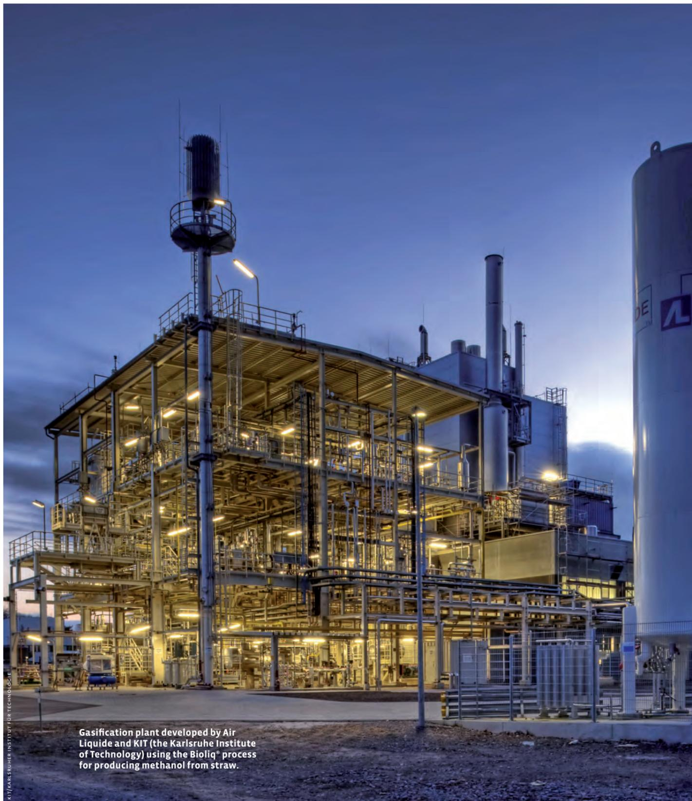
Gasification plant developed by Air Liquide and KIT (the Karlsruhe Institute of Technology) using the Bioliq® process for producing methanol from straw.
